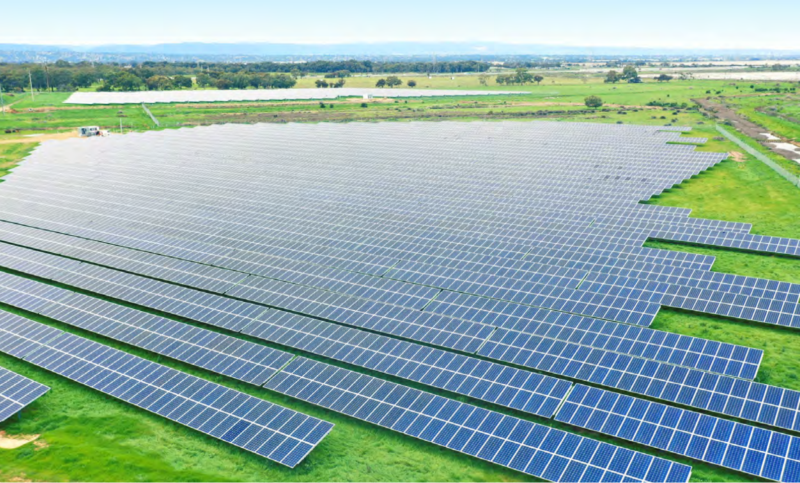
Bolivar Wastewater Treatment Plant
