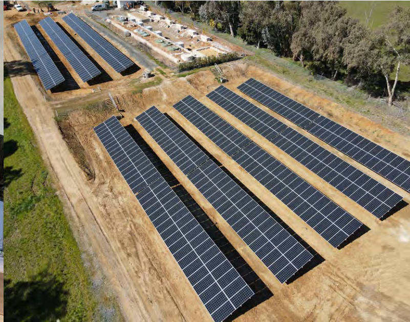
Hahndorf Wastewater Treatment Plant Reserve
