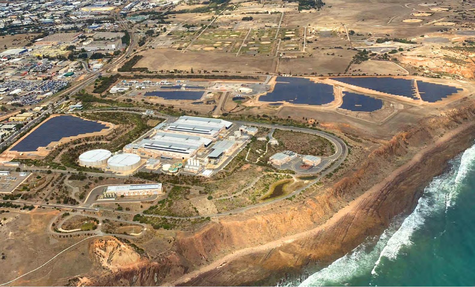
Adelaide Desalination Plant - Phase 1
