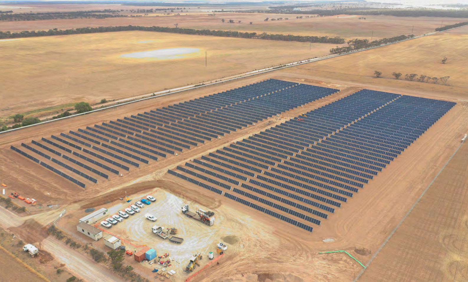
Swan Reach to Stockwell Pump Station Number 2
